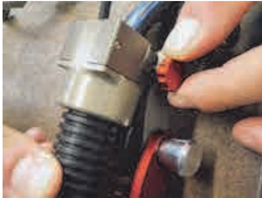
Figure 2-20 Attaching the umbilical cable to the ChainSCANNER
